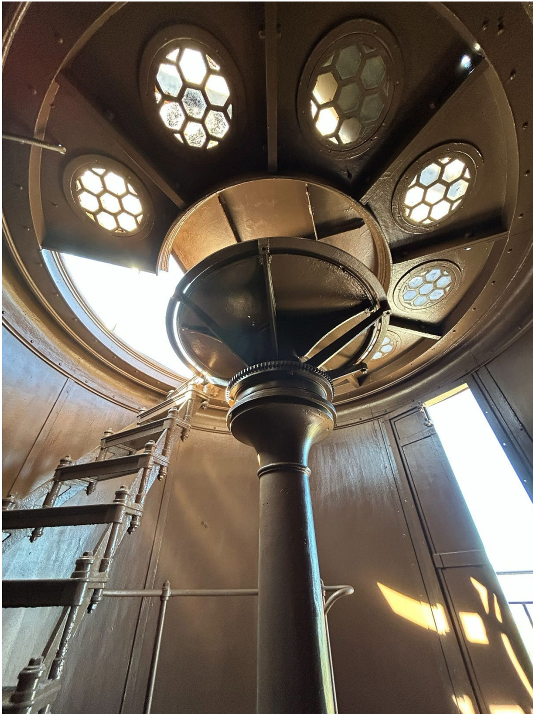
Photo 16. Eight skylights visible within the watch room ceiling which doubles as the lantern room floor. (FL_Lee_SanibelLighthouse_16).
