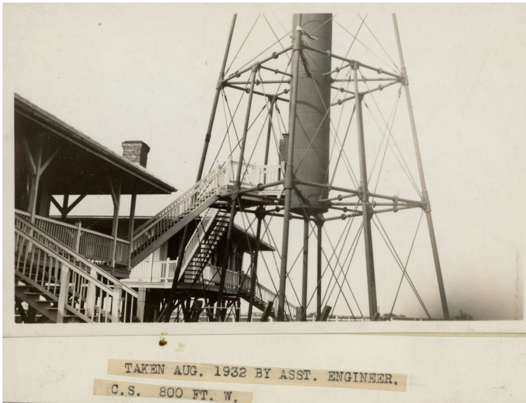
Figure 7. Historic photograph showing the original wooden stairways leading between the porches of the keepers' quarters and the entryway to the lighthouse. These stairways were removed in 1951. (Photograph No. 26-LL-Sanibel-11-1; "Sanibel Island Lt. Sta. 30 October 1941." Records of the U.S. Coast Guard, Record Group 26, Series LLS, Box Sanibel, Item #11, National Archives at College Park, College Park, MD.)
