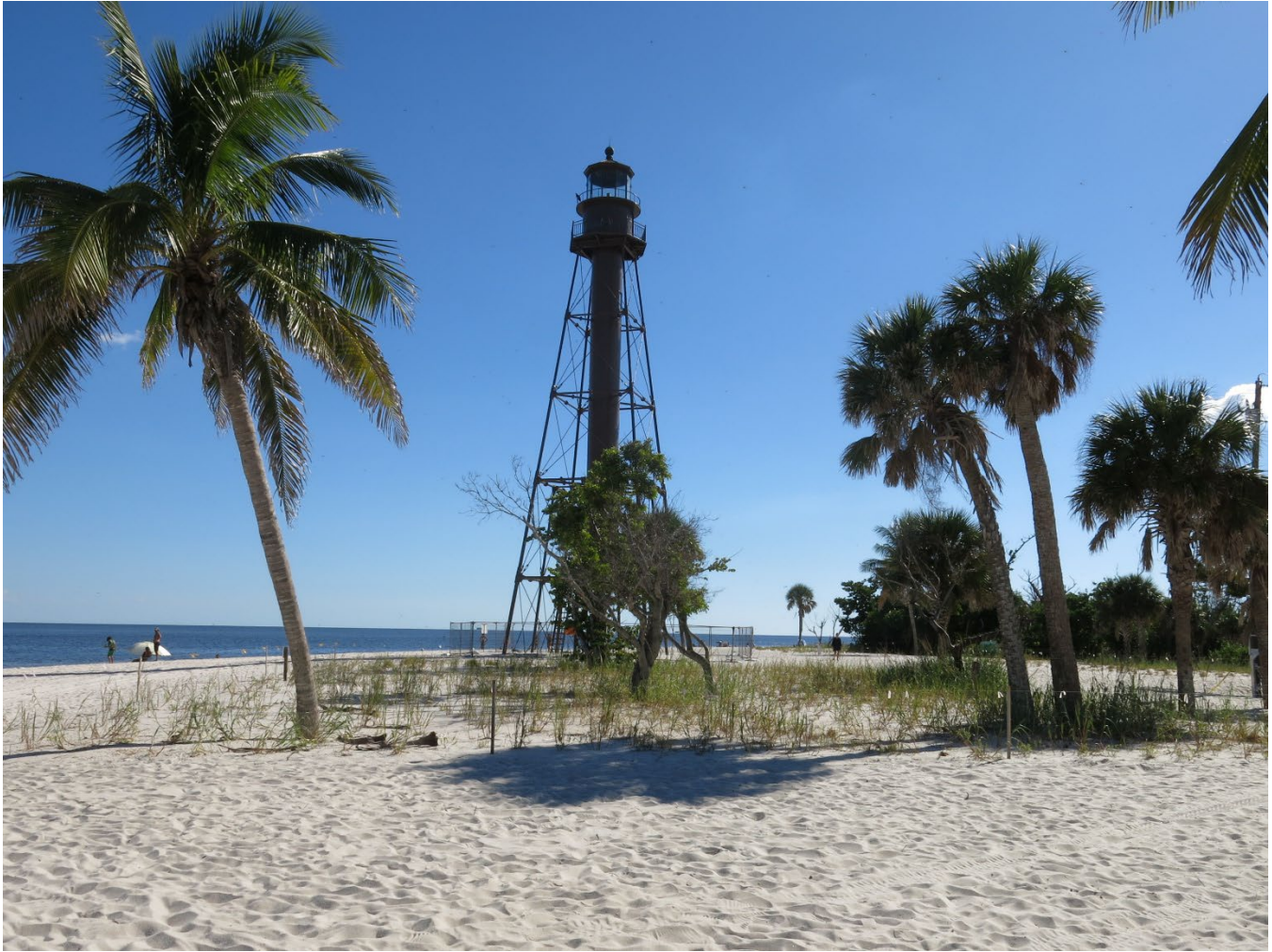
Photo 2. Setting of the Sanibel Lighthouse in 2025 following Hurricane Ian. Facing southwest. (FL_Lee_SanibelLighthouse_02).
