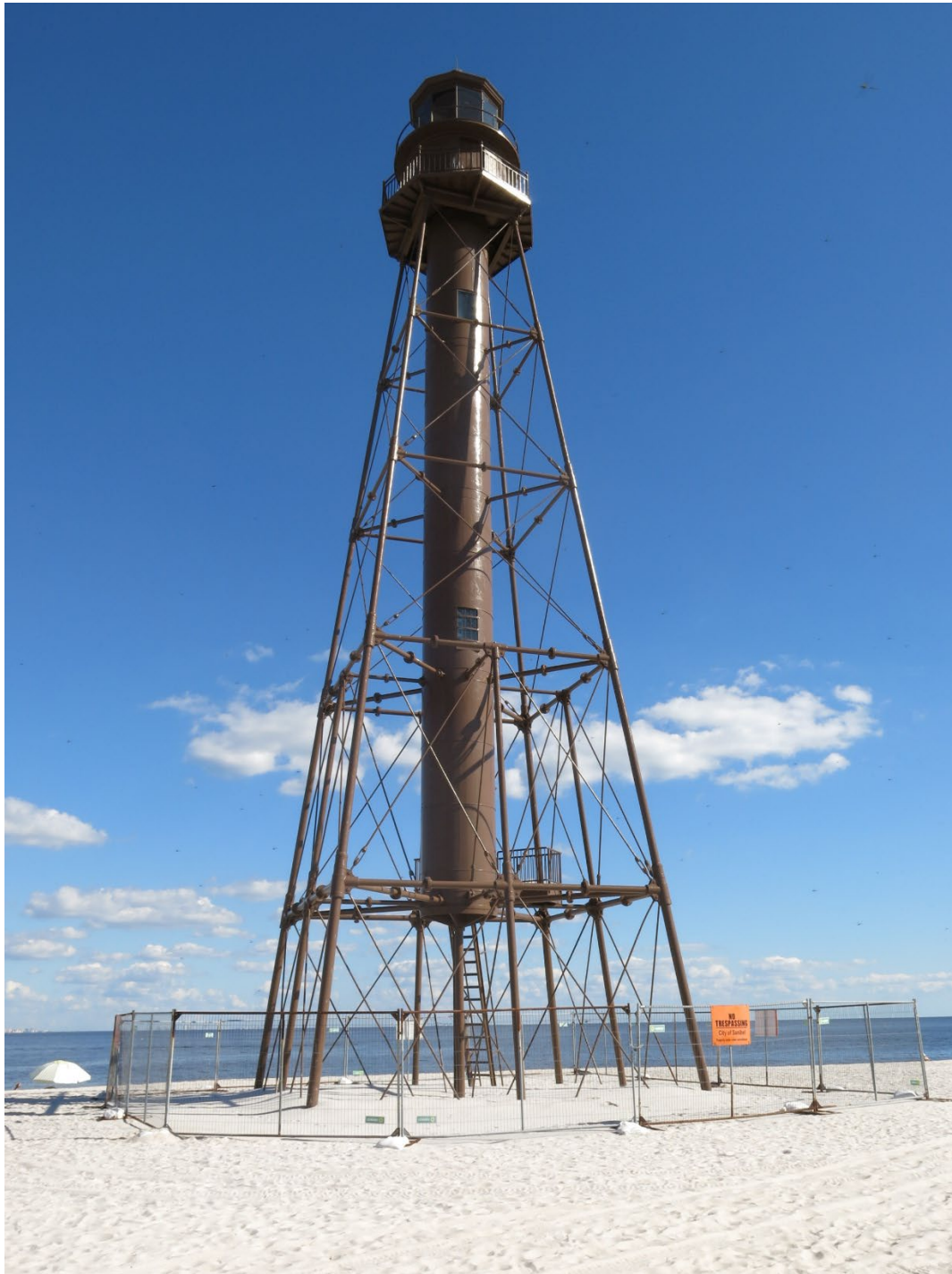
Photo 5. Exterior of the Sanibel Lighthouse, facing southeast. (FL_Lee_SanibelLighthouse_05).
