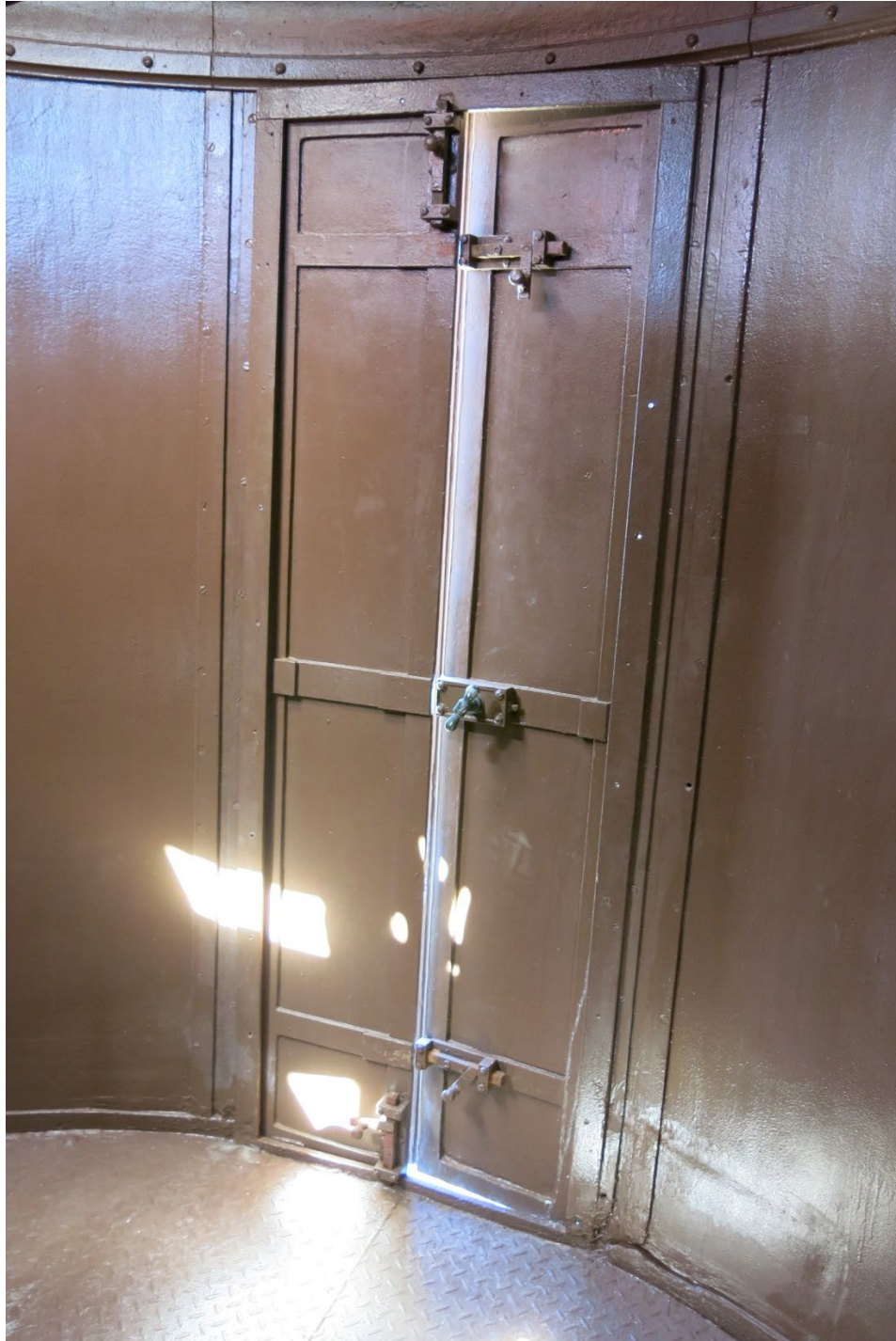
Photo 15. Interior view of the double doors leading to the gallery of the watch room. (FL_Lee_SanibelLighthouse_15).
