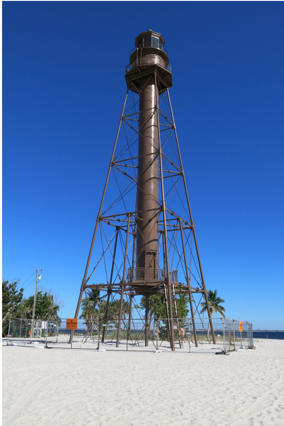
Photo 3. Exterior of the Sanibel Lighthouse, facing north. (FL_Lee_SanibelLighthouse_03).
