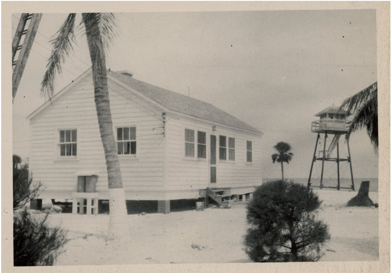
Figure 3. Historic photograph of the patrolmen quarters (left) and observation tower (right) taken September 7, 1947. (Photograph No. 26-LL-Sanibel-13-1; [SY1.1] "Sanibel Island Light Station Dwelling No. 3." Records of the U.S. Coast Guard, Record Group 26, Series LLS, Box Sanibel, Item #13, National Archives at College Park, College Park, MD.)
