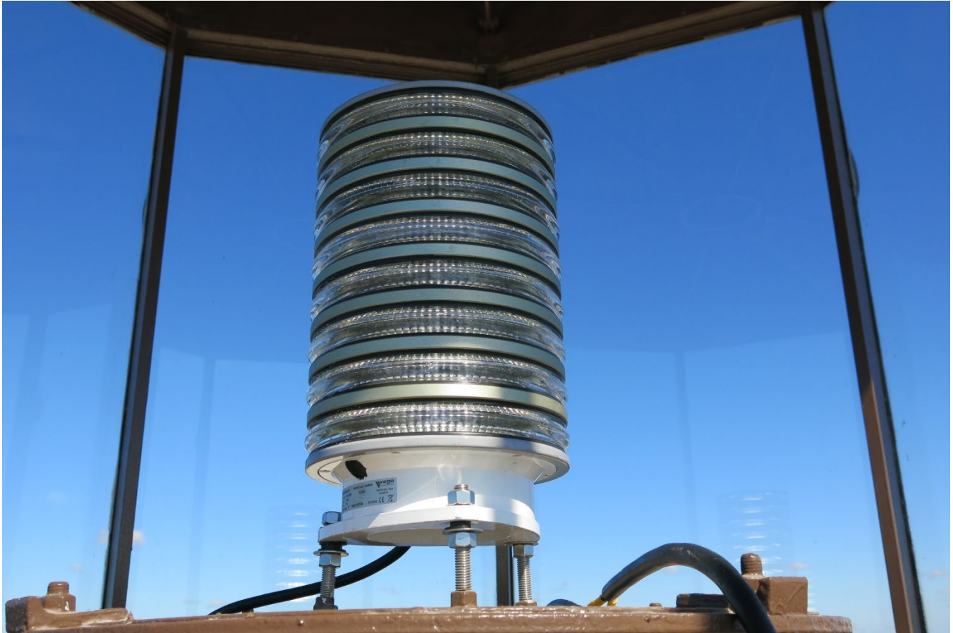
Photo 18. Non-historic LED beacon is installed within the lantern room. (FL_Lee_SanibelLighthouse_18).
