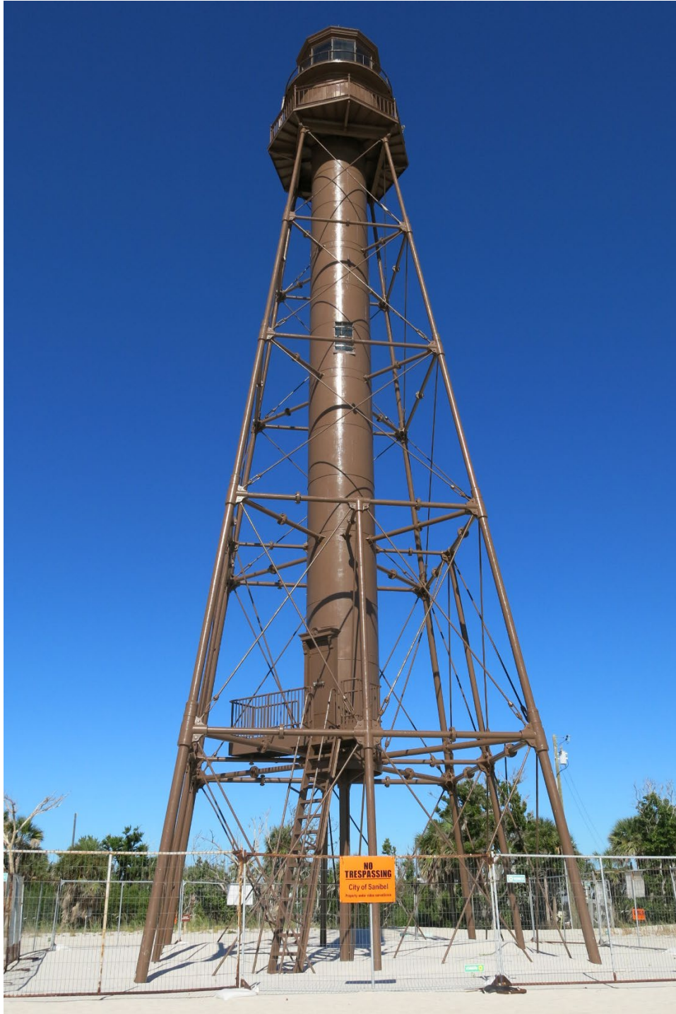
Photo 4. Exterior of the Sanibel Lighthouse, facing northwest. (FL_Lee_SanibelLighthouse_04).
