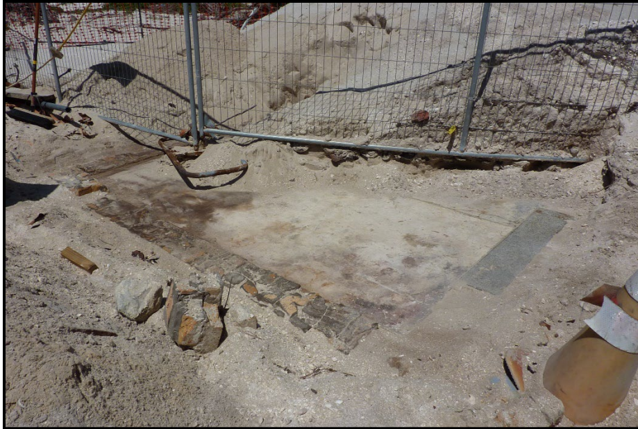
Photo 31. The partially excavated oil house foundation, looking northeast.
