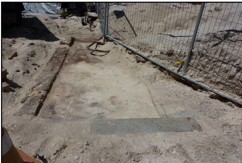
Photo 32. The partially excavated oil house foundation, looking north. Note the granite threshold in the foreground, concrete slab, and continuous brick wall around the perimeter of the slab. The right corner and wall are covered with piled sand being utilized for erosion control/shore reconstruction and the temporary metal fencing separating Lighthouse Beach Park from the construction site.
