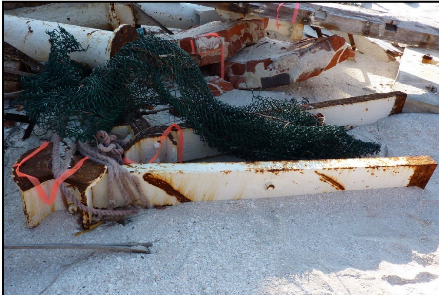
Photo 25. Two bracketed metal girders located within the debris pile (Group No. 6 and 7).
