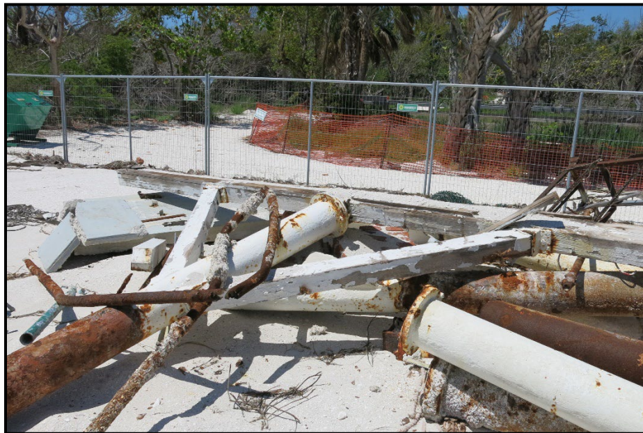
Photo 15. Wooden girder with intact metal support post and wooden brackets.
