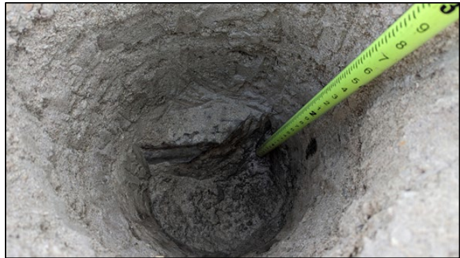
Photo 5. ST 1 with foundation.
