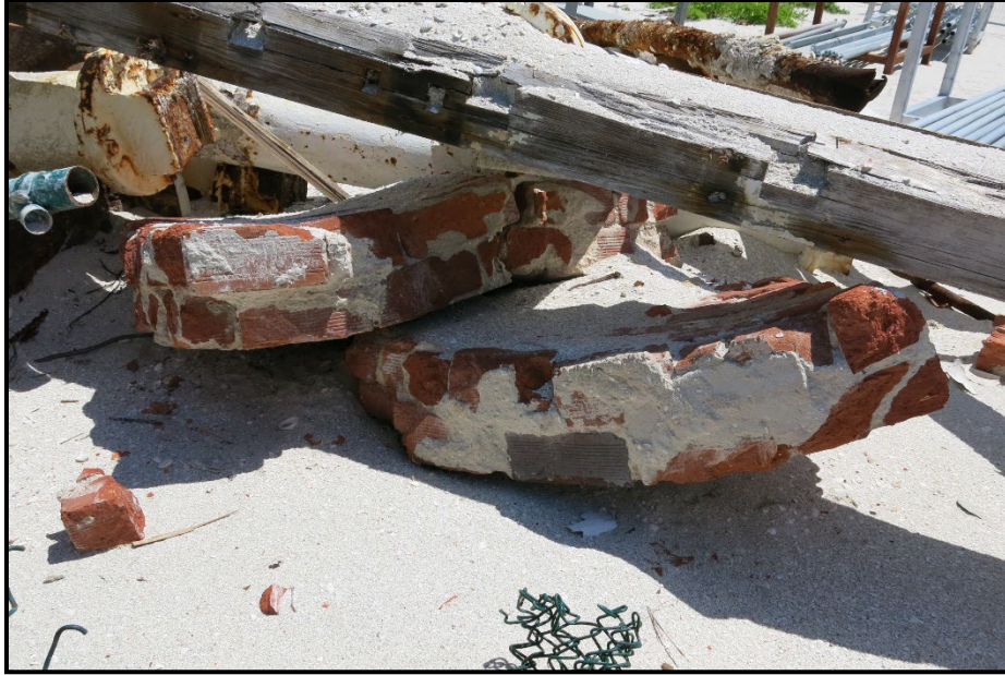
Photo 16. Two curved segments of the cistern walls comprised of striated face brick constructed two wythes thick with intact mortar.
