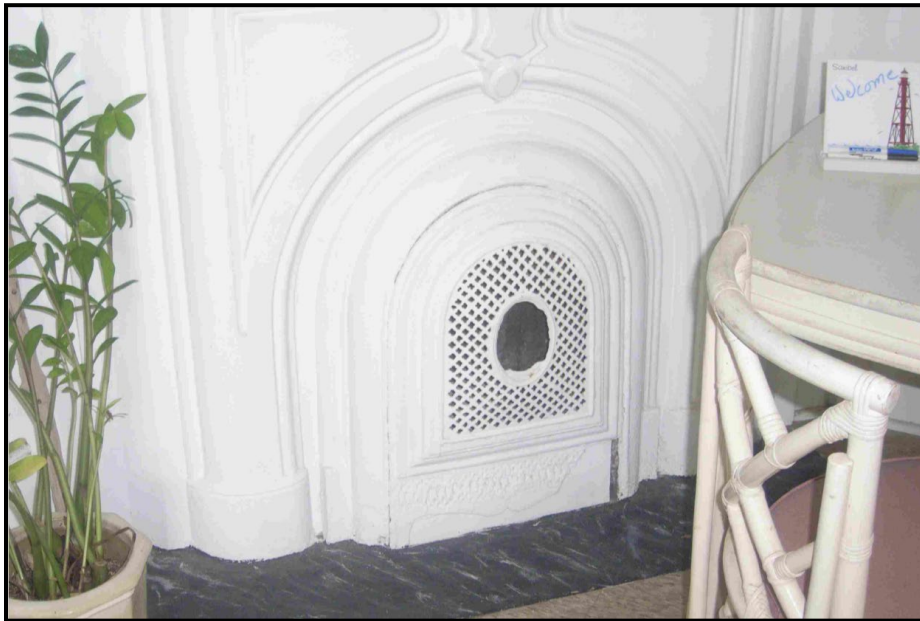
Photo 24. A photograph of one of the Keepers' Quarters coal burning fireplaces. Note the decorative cast iron surround (painted white) and slate hearth (FMSF n.d.).
