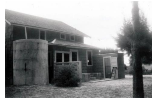
Cistern to collect rainwater attached to Powell Home, 1939 (Powell Family Collection)
