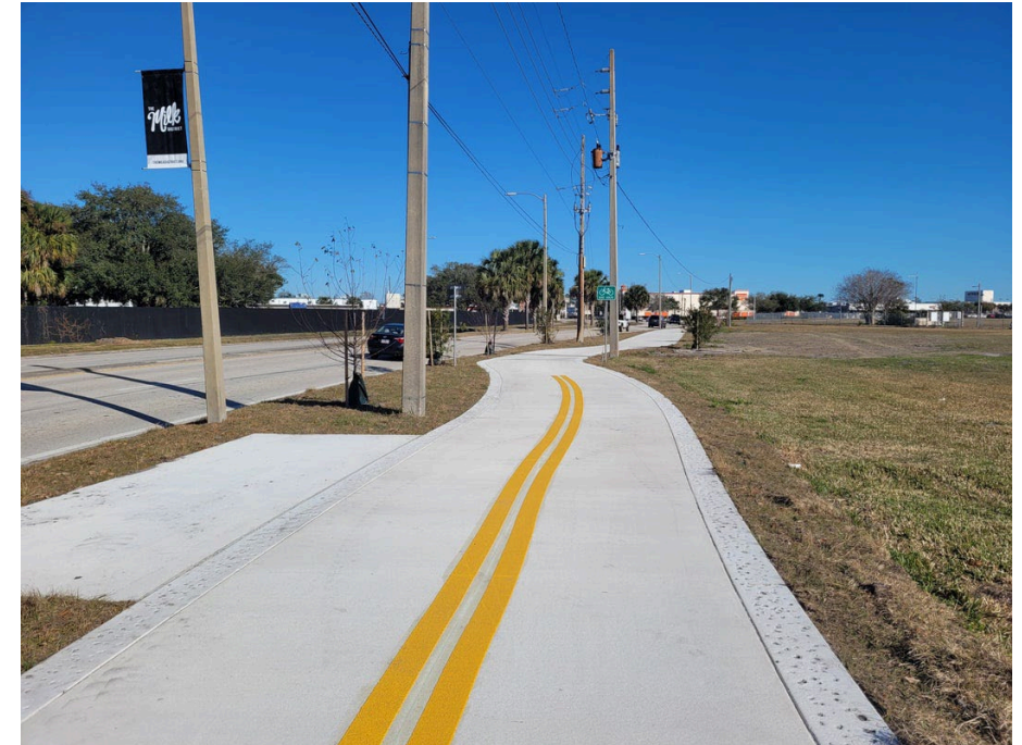
Source: Maguire Boulevard, Orlando. Kittelson & Associates, Inc.
