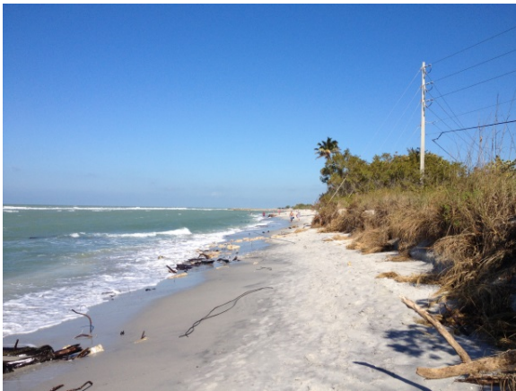
Figure 4: Photo of erosion south of Blind Pass beach showing proximity of erosion to power pole guy-wires 2/10/15
