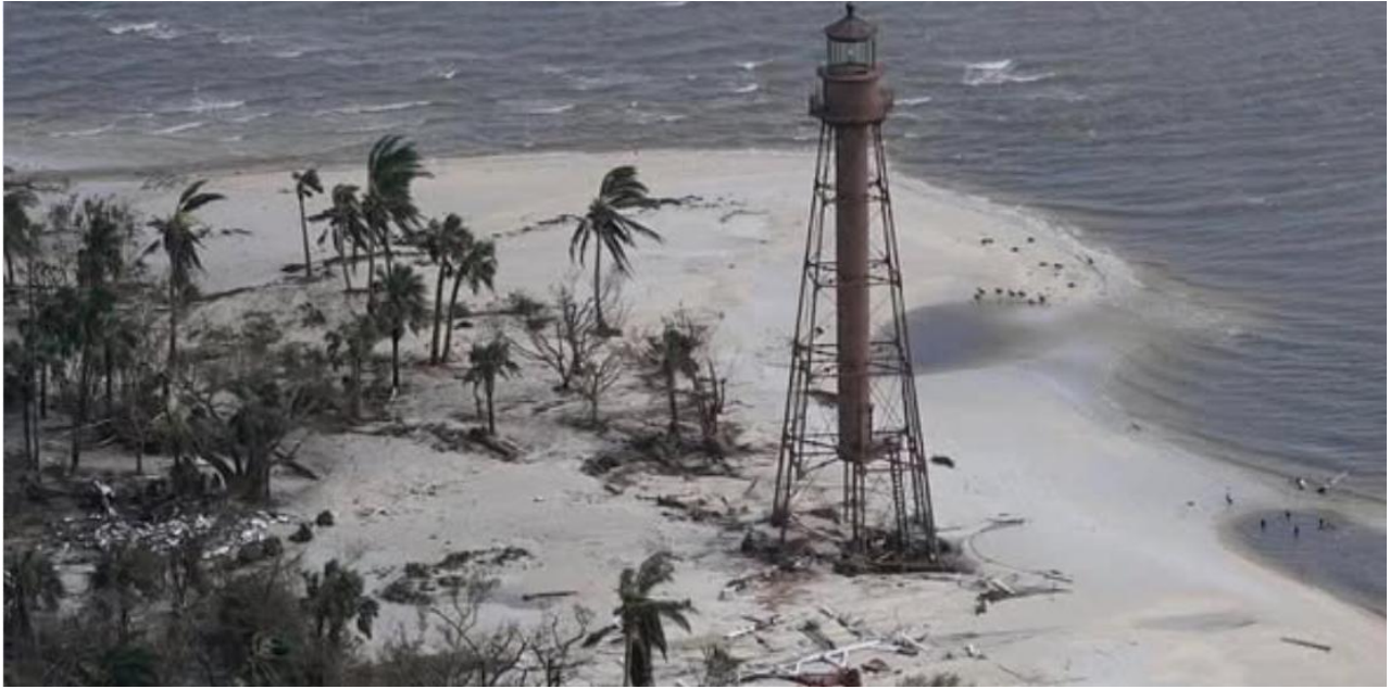
Post Hurricane Ian 2022
