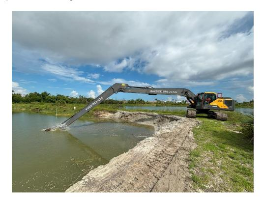
A cellular geotechnical grind will be placed on the slopes and filled will soil dredged from Pond 3. Once stabilized, vegetation will be planted to further reduce the risk of future slope failure.
