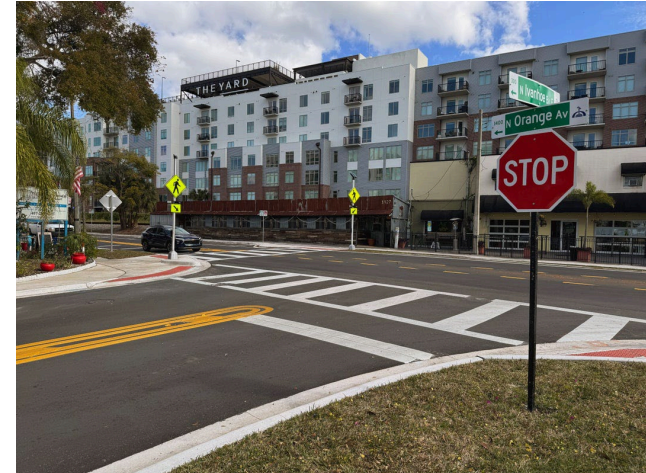
Source: N Ivanhoe Blvd and N Orange Ave, Orlando. Kittelson & Associates, Inc.
