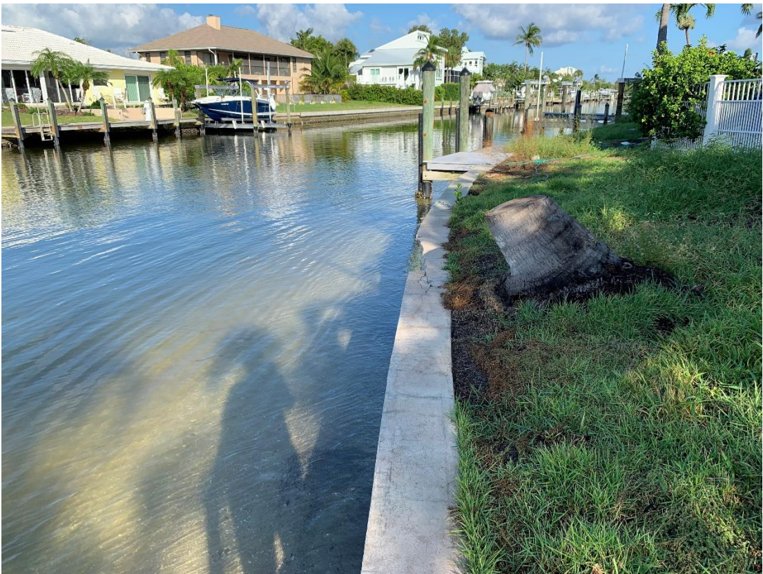
Figure 1. Seawall looking west
