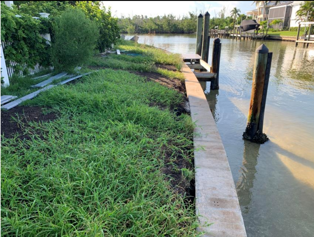
Figure 2. Seawall looking west
