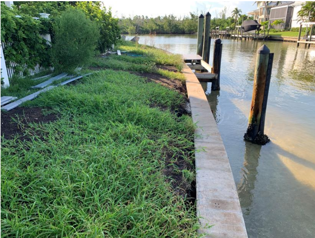
Figure 5. Seawall looking east
