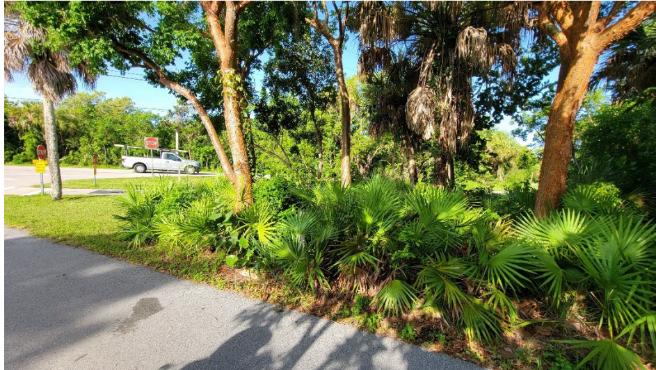
Figure 10. Vegetation Obstructing View at Parking Area Exit Facing West Towards Path
