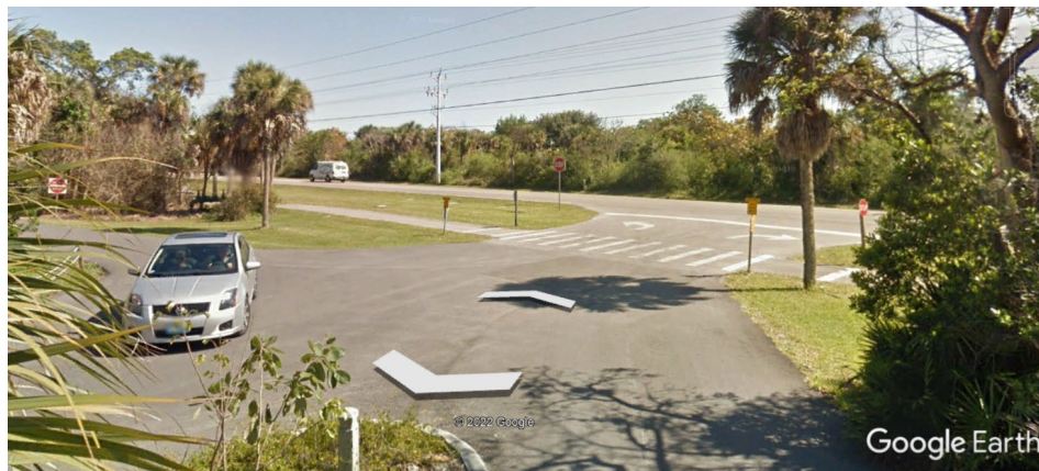
Figure 9. Vegetation Obstructing View of Shared-Use Path at Parking Area Exit
