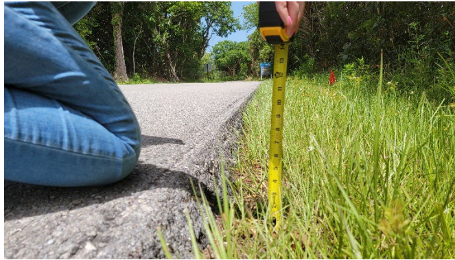
Figure 6. Refuge Entrance and Edge of Pavement Drop Off
