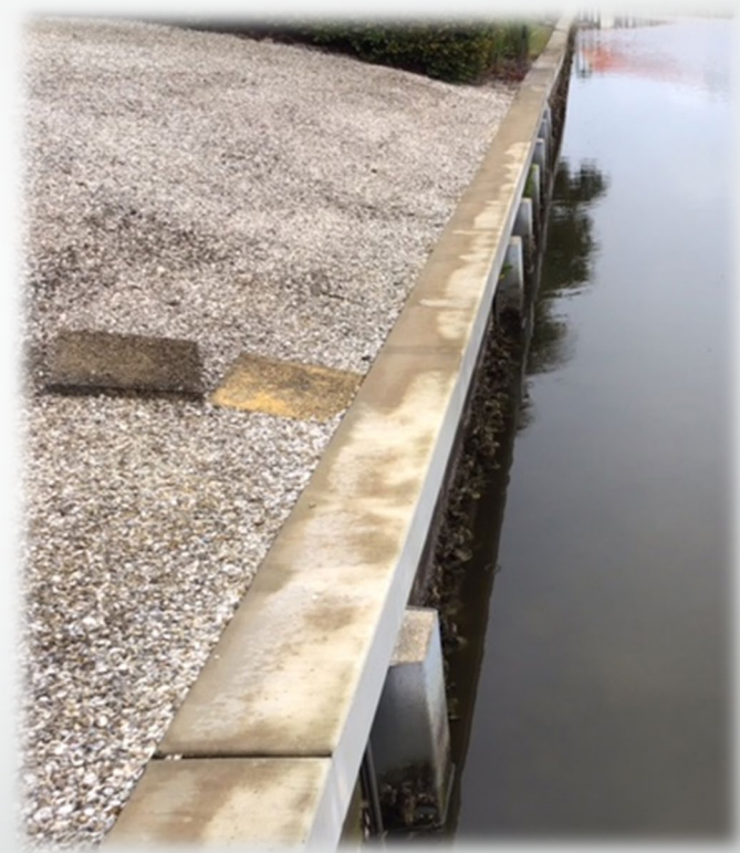
Seawall Cap and Reinforcement Pilings Shell Harbor
